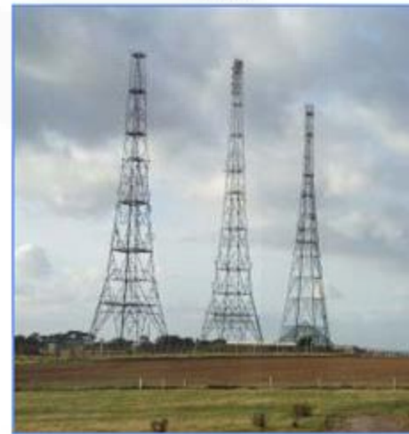
Sept 2006 Photograph of Three Chain Home Transmit Towers, near Dover
